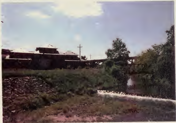
Fig. 15 The mouth of the French Creek near its junction with the Schuylkill River at the site of the former Phoenix Iron Works. Photograph by the author, 1994.
